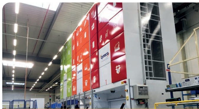
Fire protection system integration
